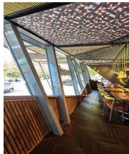
is assembled and glazed onsite, offers the slimmest and most consistent sightlines once installed – typically 50 mm for both the mullion and transom. It also easily caters for staggered transom and mullion options if required.
