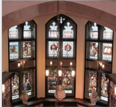
They all had single glazed openings which could not prevent draughts efficiently or keep the noise out. To complement the interior decor and leaded casings, the timber sub frames and secondary glazing profiles were colour coated in 9005 Jet Black Matt.
