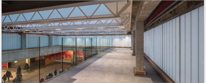
protection, maintaining privacy for the residents and controlling light pollution, while bathing the interior with diffused daylighting, regardless of the weather. The panels are lightweight but very durable with excellent resistance to impact and scratching. They are also vandal resistant with good protection against windborne debris.
