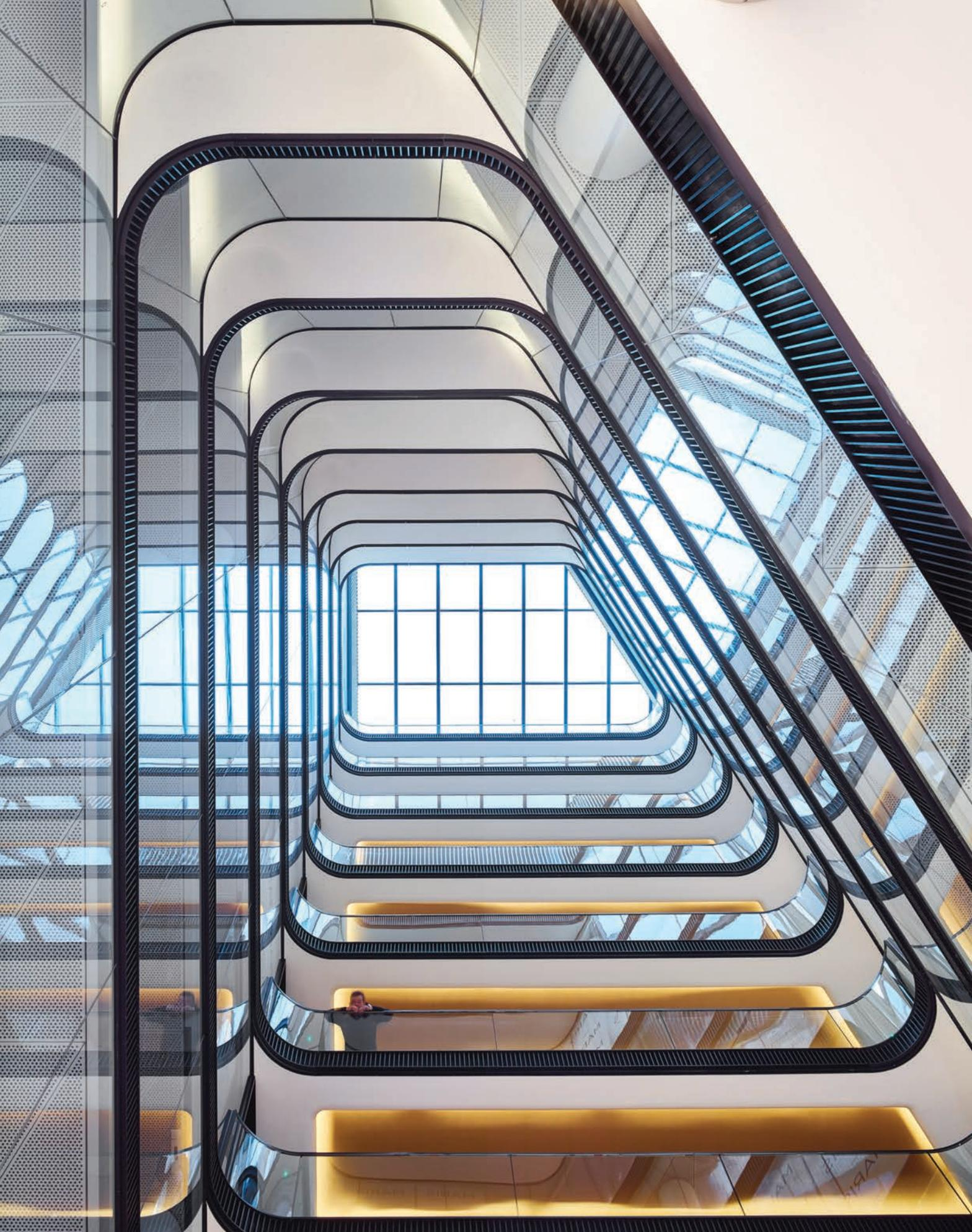
building's interiors, as well as providing an inspiring entrance to users as they approach the reception. "Laminated safety glass was used for the atrium and towards the nose of the building the atrium's corners are curved, allowing the softness of art-deco and art-modern to be played out," says McRae.
