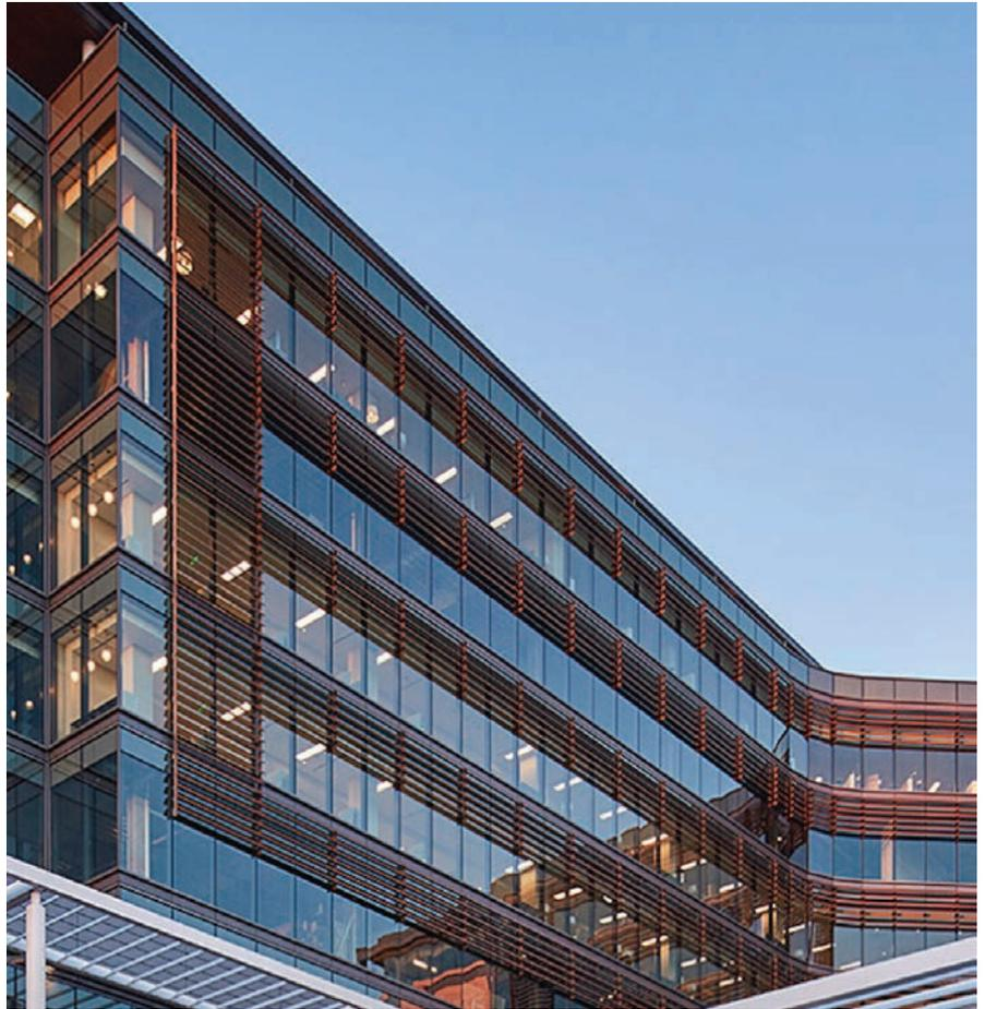
Jacksonville, USA, adopted an holistic approach to the building design, using natural materials extensively. It was found that where wood was impractical to use, the designers retained the overall natural look on aluminium aerofoil blades, providing a credible substitute.
