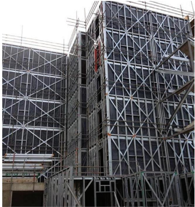
**We have in recent years seen cold rolled replacing hot rolled steel in areas such as small to medium portal-framed and beam and column structures within the retail, commercial, agricultural and leisure industries**
