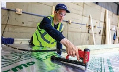
Thermo Extreme helps deliver low overall U-values when the foil faces into an unventilated airspace, achieving an aged thermal resistance R-value of 0.77m<sup>2</sup>K/W, incorporating printed branding.
